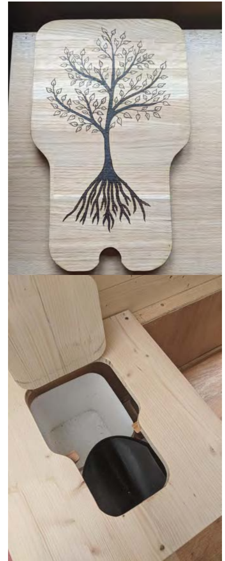
Above - Composting toilet interior, with urine separator (black) and solids box (white), and a tree pyrographed onto the lid.
