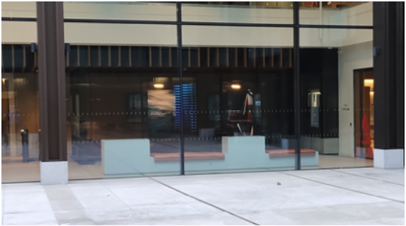
In 2018, the Fruit and Wool Exchange was redeveloped, with only the façade facing Brushfield Street surviving. Dorset Street was obliterated, and the site of Mary Kelly's murder is behind this glass, in the soulless foyer of a modern office block.
