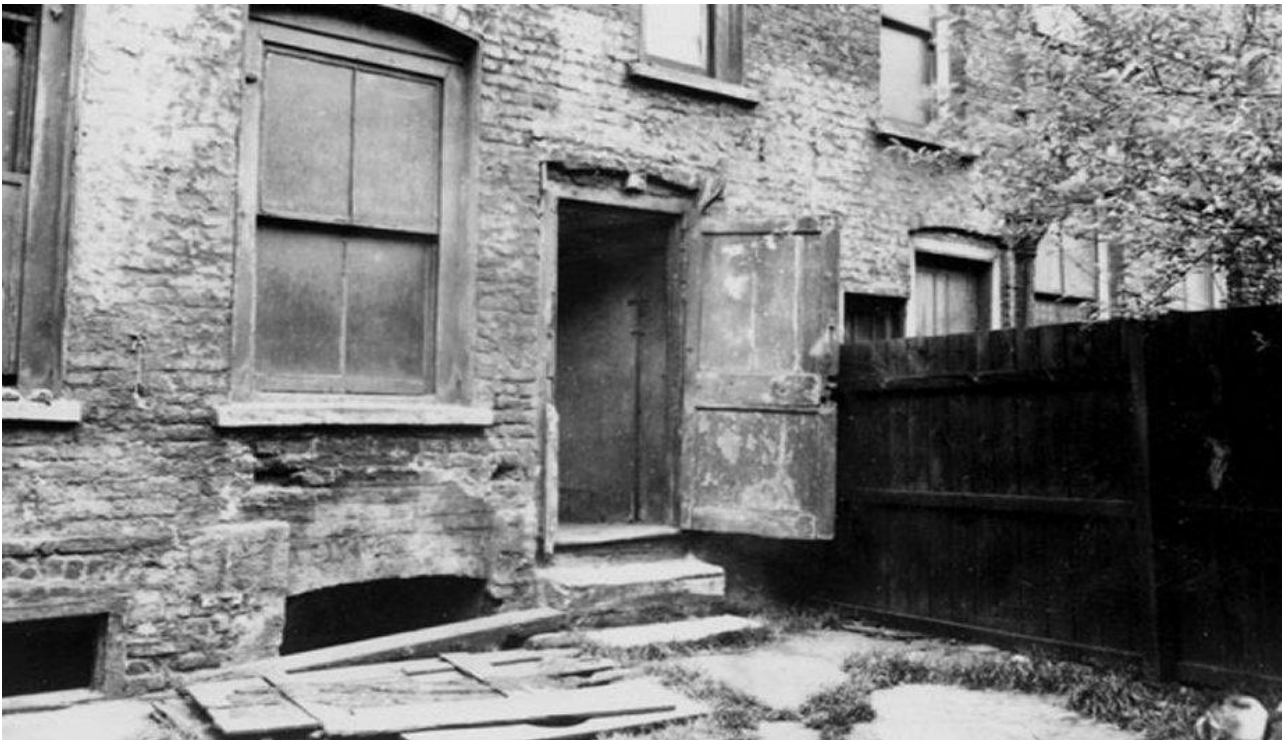
The backyard of 29 Hanbury Street as it was. Chapman's body was found by the fence on the right. (Source: Wikimedia Commons.)
